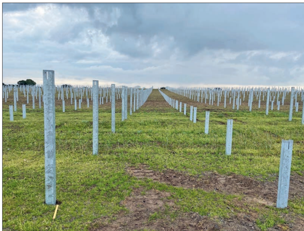
Figure 6. C-shaped metal posts onto which the solar panels will be fastened. Photo: Niclas Horn, Better Energy.
